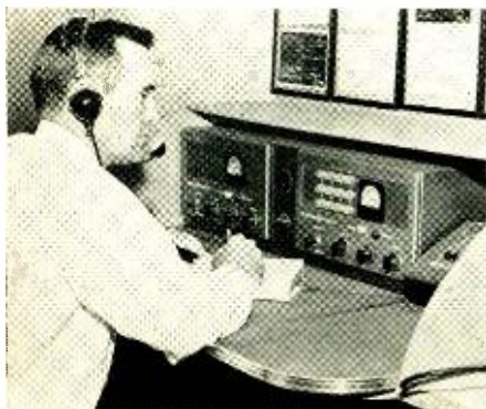
Close-up of operator at controls of the master console in the truck trailer communications center.
